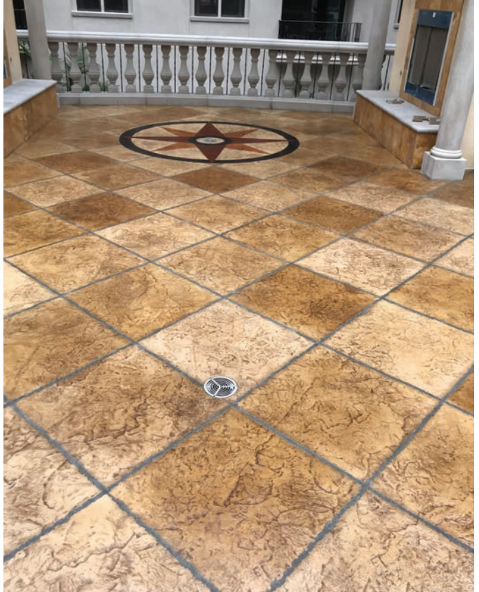
Roman Slate / Saw-Cuts Cappuccino Color Hardener / Desert Tan Antique Release / Acid Stain (diluted)
