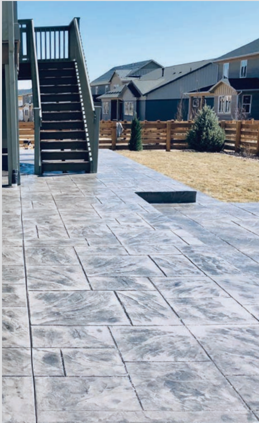
Large Ashlar Cut Slate Stone Gray Color Hardener / Medium Gray Antique Release
